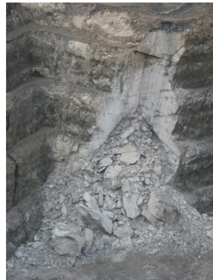
Figure 1 Wedge failure on a bullnose
